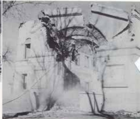
Old Hadley being torn down. Images are from the 1958 yearbook.
