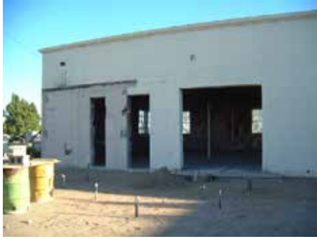
Northern exterior wall of the kitchen area.
