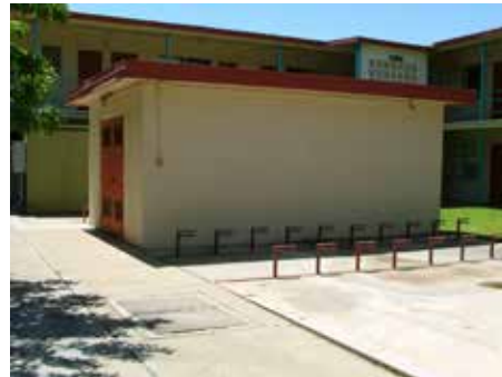
Pump House located in the eastern courtyard of the "H."
