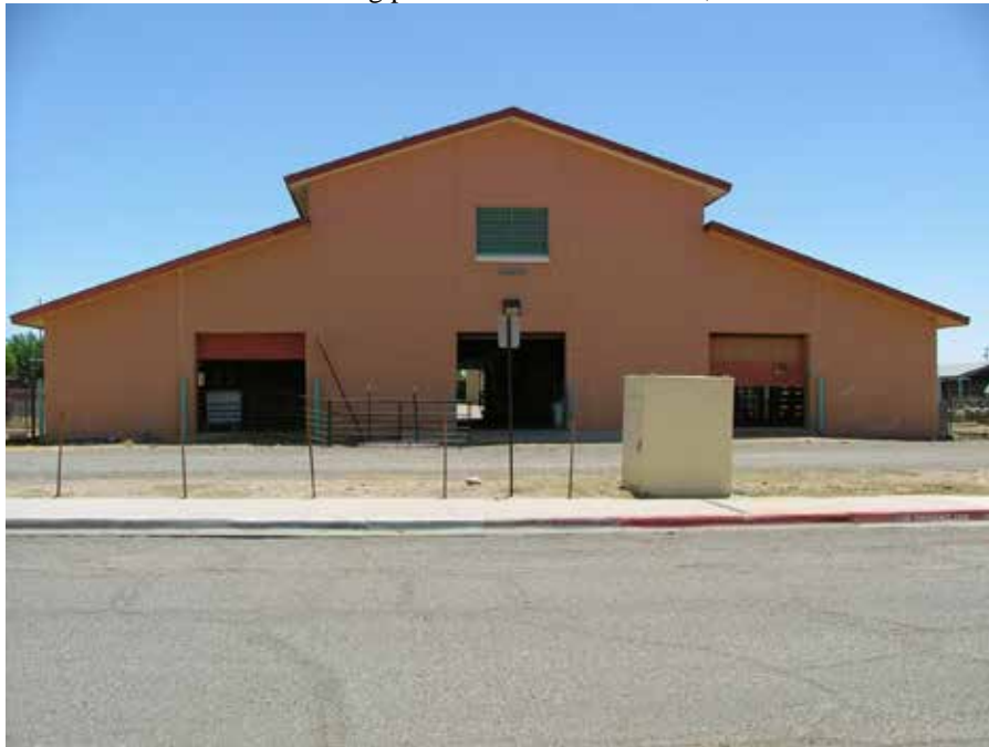
North side of the barn.
