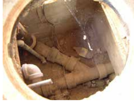
Old pipes under the flooring.
