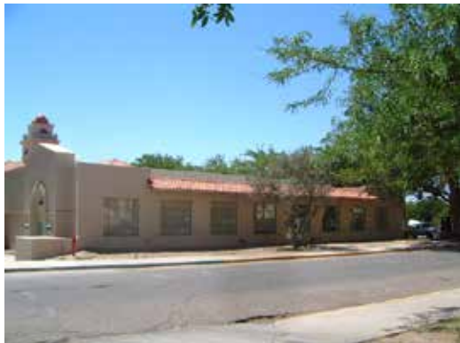
2001 - Annex East Side
