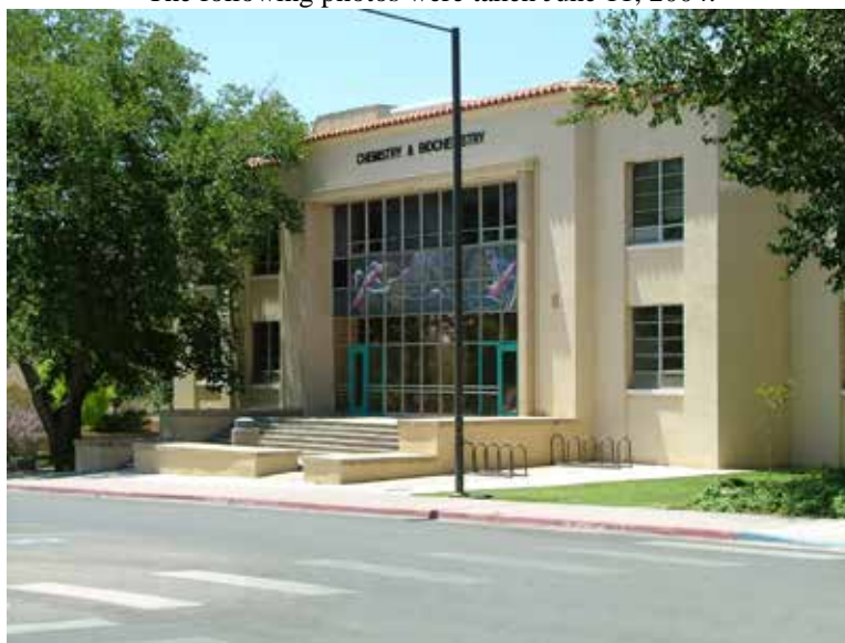
Main entrance to the Chemistry Building.
