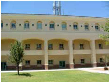
South side of the northwest wing.
