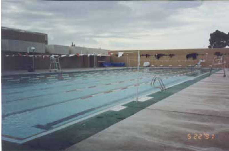
Photo of building #322 taken May 22, 1991. This is the way the pool looked prior to the 2002 renovation.
