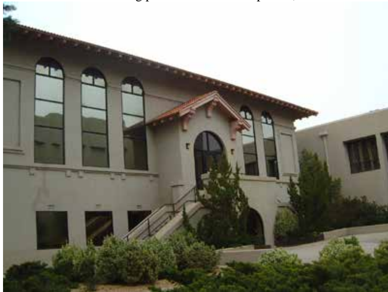
South entrance to the "Gymnasium."
