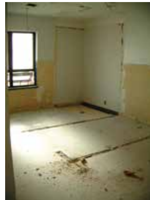
Bathroom at the end of the north wing.
