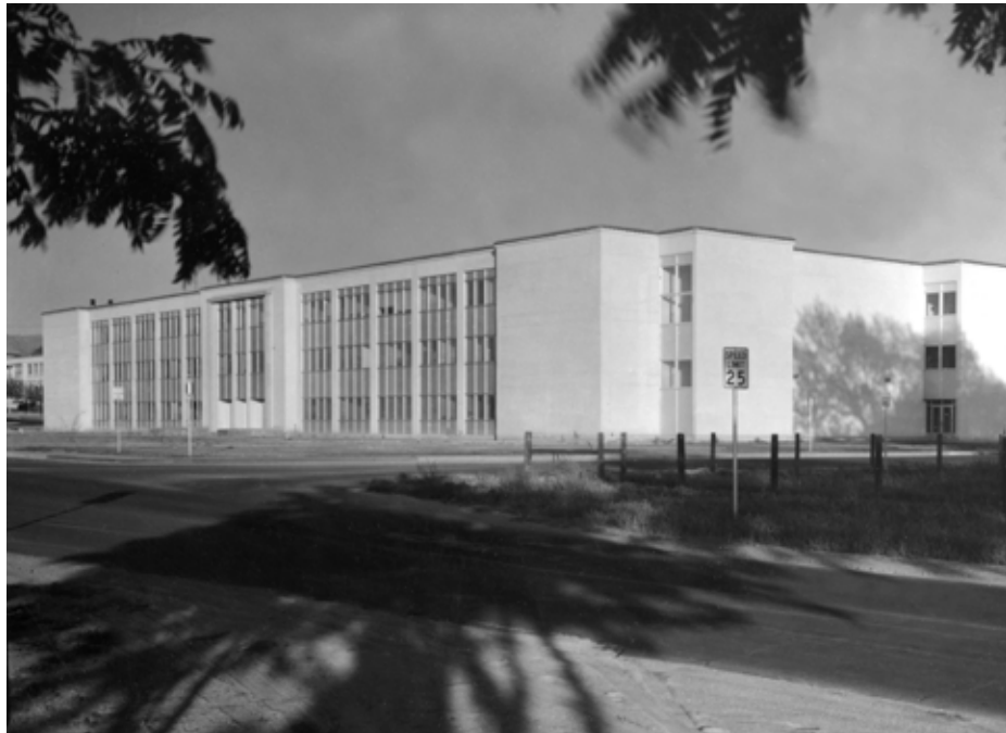
Photo of the north side of the building, circa 1963. Photo courtesy of University Archives.
