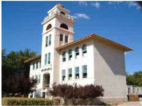
2001 – Demolition For Renovation
