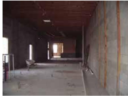
1968 addition looking south with new concrete floor.
