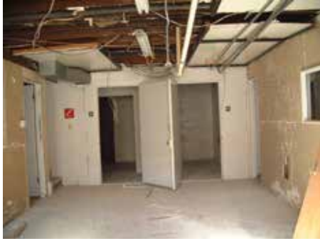
(Left) Basement main room.
