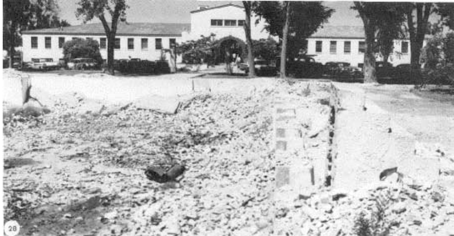
Hadley Hall is pictured in the background of this photo of the remains of Old Hadley Hall after it was demolished. Photo is from the 1958 yearbook.
