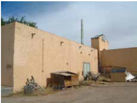
West side of the building.
