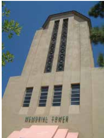
Top of front of the tower.
