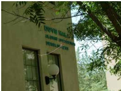
Old signage located on the north east corner of the building that was not replaced when the rest of the buildings on campus received new brown lettering. Photo taken June 11, 2004.
