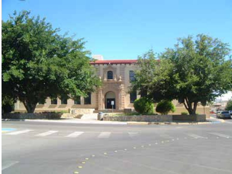
North side of Foster Hall. Photo taken July 14, 2004.
