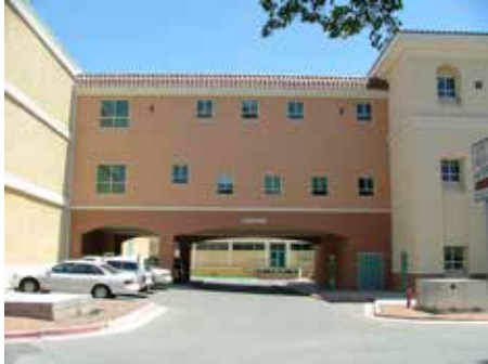
Connection between the northeast and the northwest wings.
