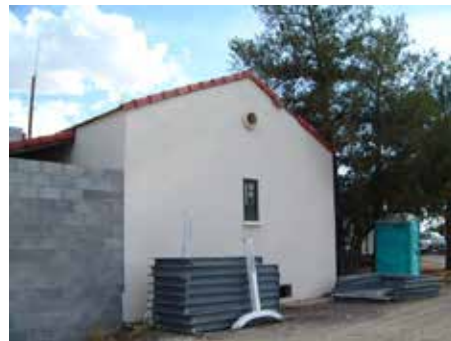
Northern exterior wall. The cinderblock attached to it is new construction.
