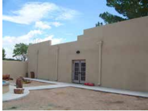
The northern exterior of the east wing.
