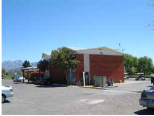
Northwest side of the building.
