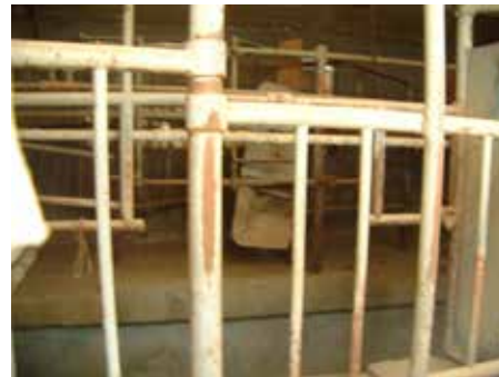
View inside room 9 through the window shown in the previous photo.
