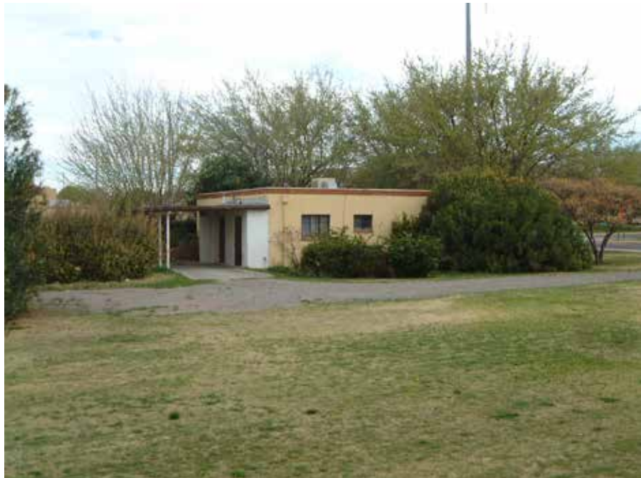
Back or west side of the building.
