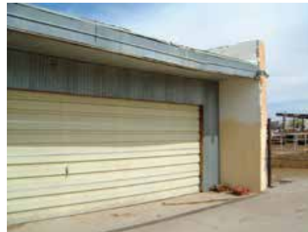
View of the west exterior of room 20.
