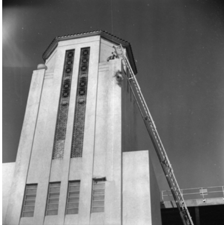
Photo of the southwest urn being pushed off of the tower circa late 1960's. This was done to install an antenna in its place. Photo courtesy of University Archives.
