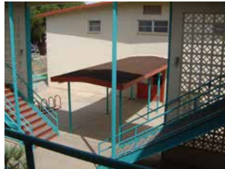
South entrance to the "600" building.
