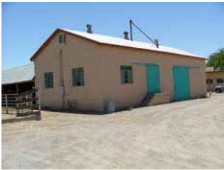
Photo of the northeast side of the building taken June 11, 2004.
