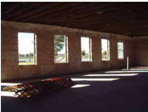
South exterior wall of the main dining hall.
