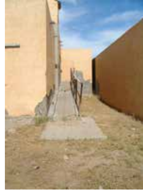
Ramp on the south side of the storage room.
