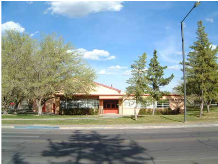
Photo of Era Rentfrow Gym taken March 24, 2004.
