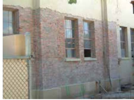
Brick on the east side of the building.
