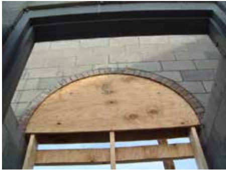
Arch for the new east entrance.
