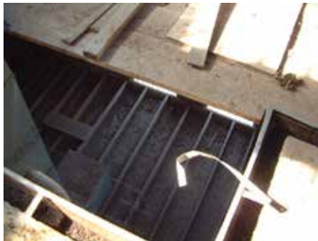
View of the roof of the 3 rd floor's west room.
