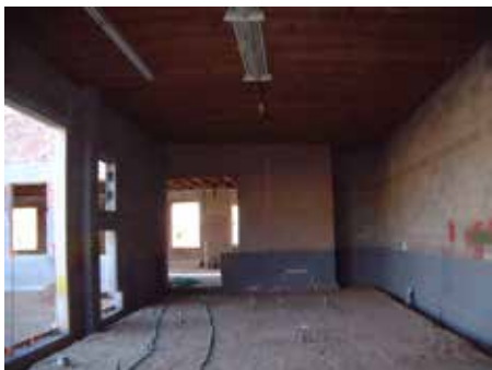
Looking south in the 1968 addition.
