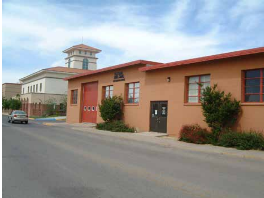
Photo of the front of the Tejada Building taken April 27, 2004.
