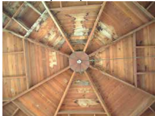
Roof of the Tower.
