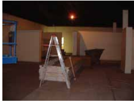
Art Gallery Construction.
