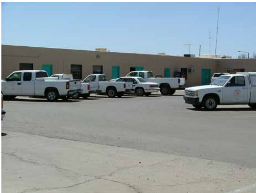
West wing of the shops building is home to other shops such as the electrician's shop and the sign shop. Photo taken June 11, 2004.
