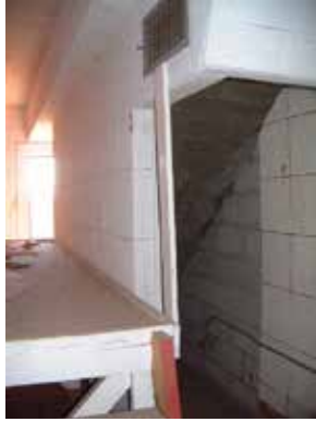
Storage room under the stairs leading to the 4 th floor.
