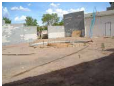
New court yard construction.
