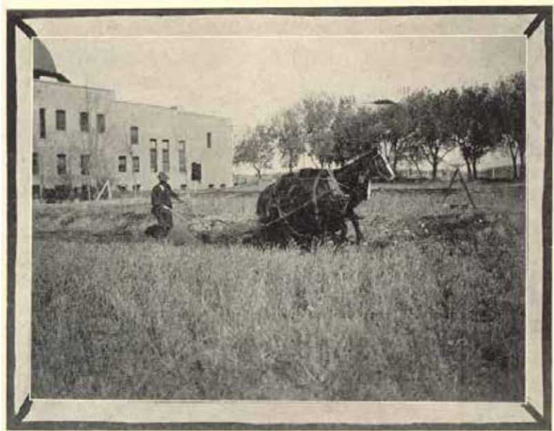
Breaking the Ground for the New Library
