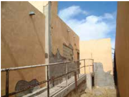
Looking at the south side of the storage room.
