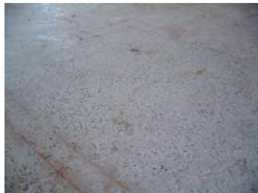
The original Terrazzo flooring.
