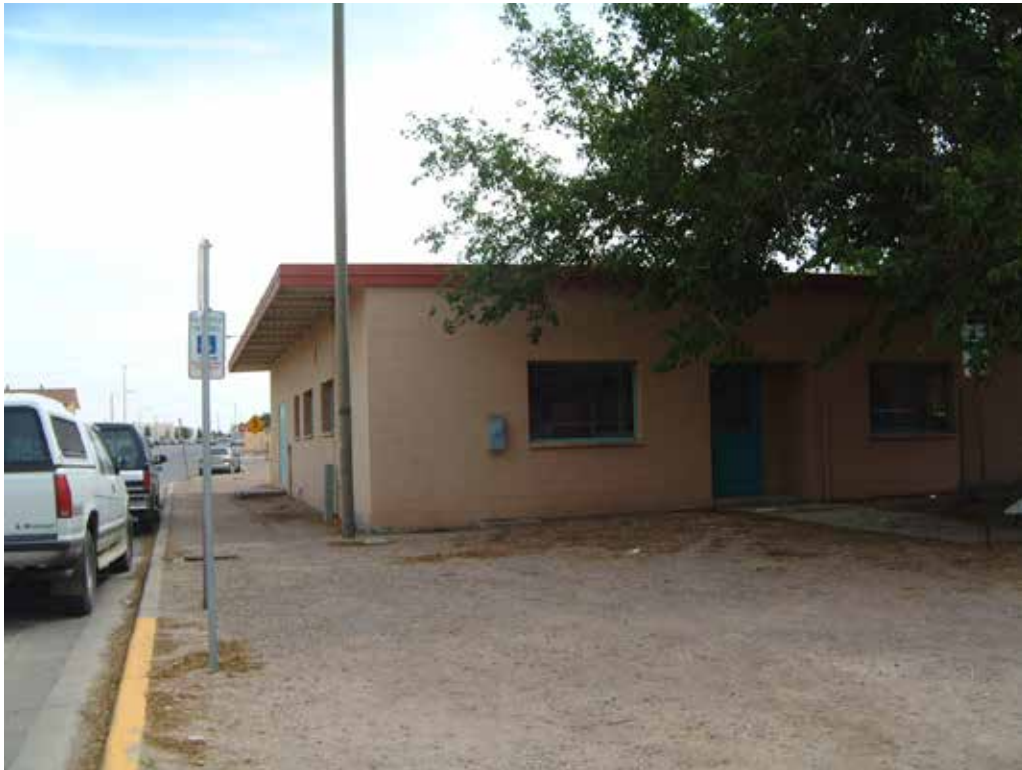
Northeast side of the building. Photo taken April 27, 2004.
