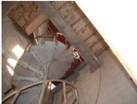
Spiral stairs to the 5 th and 6 th floors.
