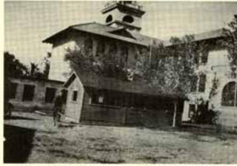
The Radio Shack, KOB's original home. (R. W. Stewart photo)
