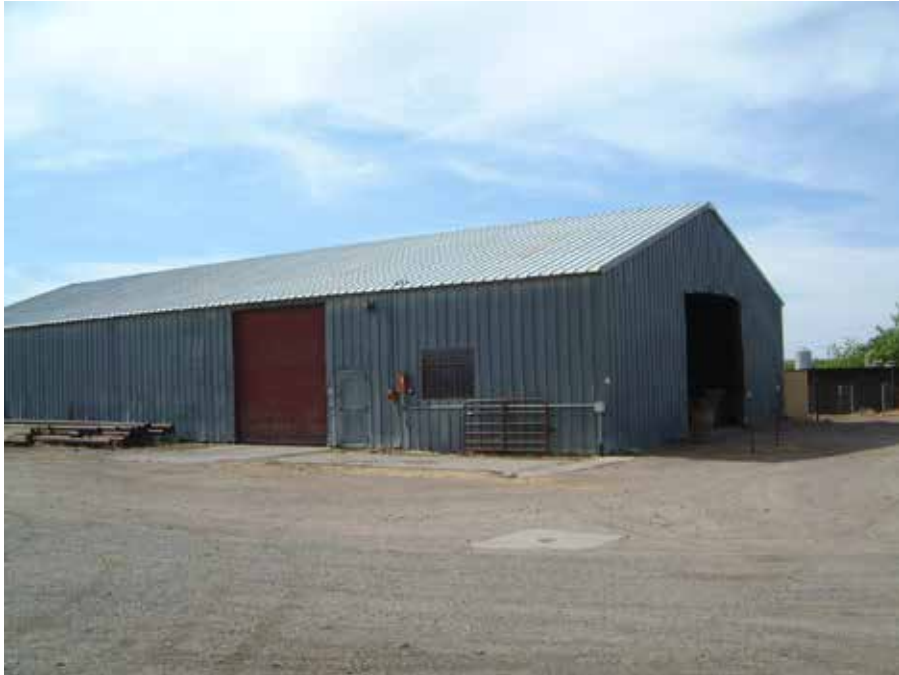
Photo of the southeast side of the building taken April 27, 2004.
