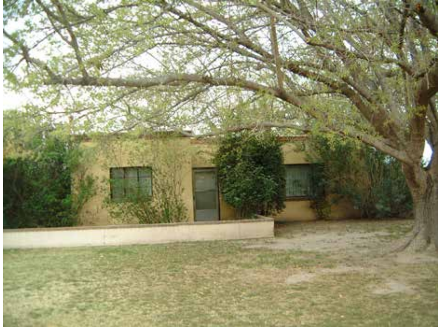
Front or east side of the building.
