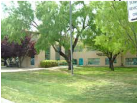
East entrance to building.
