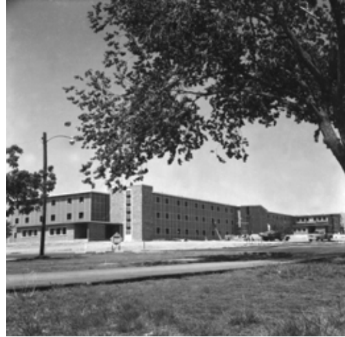
Near the completion of construction.
