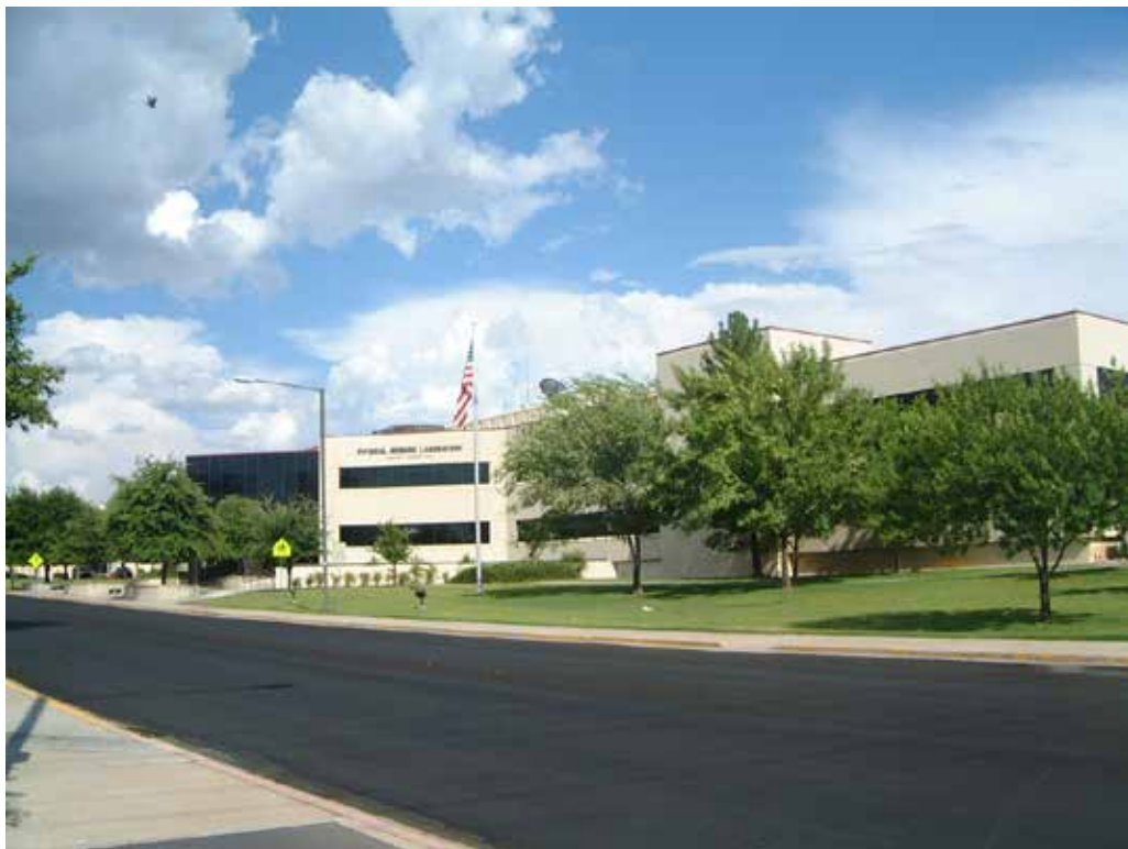
Photo of the north side of PSL taken July 11, 2004.
