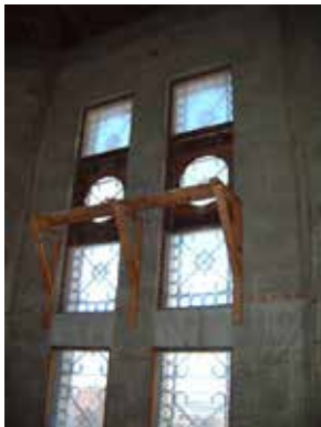
Inside of the tower windows.
