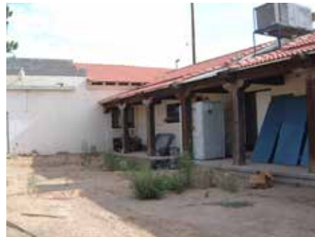
Porch located on the west side of the north wing.
