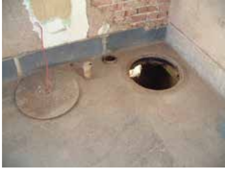
Manhole access to chases under the concrete sub-floor.
