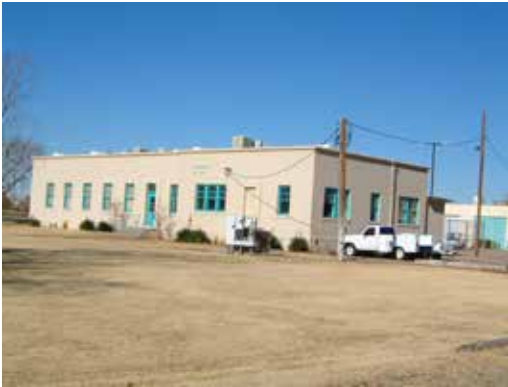
(Left) June 21, 2001 Prior to any renovation work.
