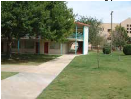
Northeast wing east stairs.
