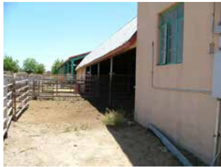
Photo of the west side of the building taken June 11, 2004.
