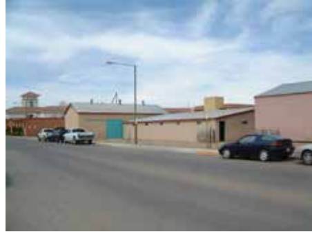
Photo of the southwest side of the building taken April 27, 2004.
