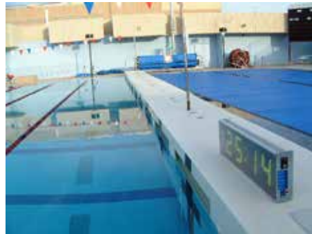
Divider that separates the diving section of the pool from the main part of the pool.
