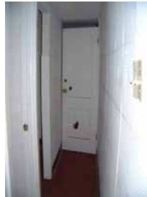
4 th floor hallway.
