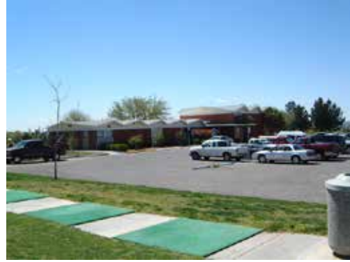
North side of the building.
