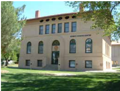
The front of the building after the completion of the renovation.
