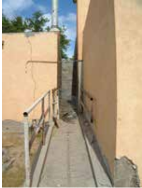
Ramp on the north side of the storage room.
