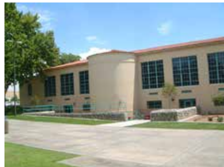
North side of Milton Hall that was renovated in the spring of 2004.
