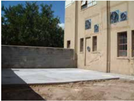
Location for the exhaust system.
