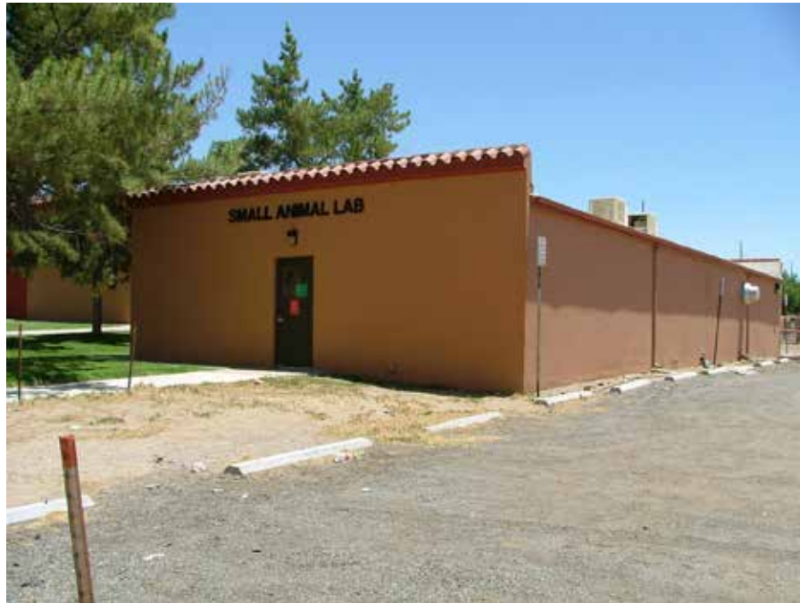
North side of the building. Photo taken June 11, 2004.
