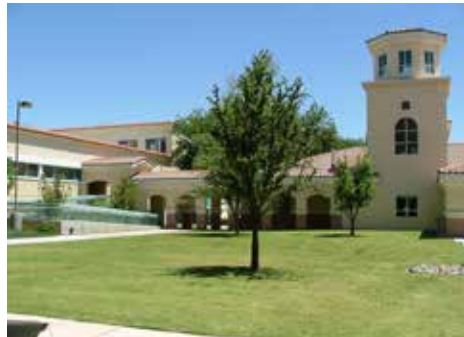
Connection between the last addition (southeast wing), and the original part of the building.
