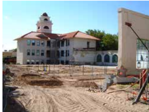
2001 – Demolition For Renovation
