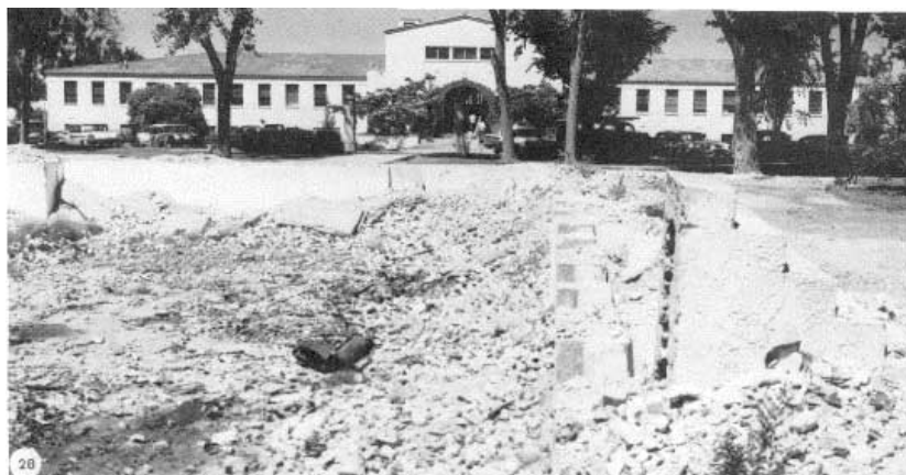
Photo from the 1958 yearbook, shows all that remained of Old Hadley Hall after its demolition. The new administration building (Hadley Hall) sits in the background.
