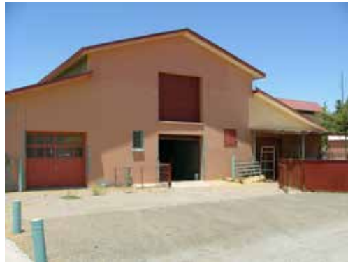
South side of the Sheep Barn.
