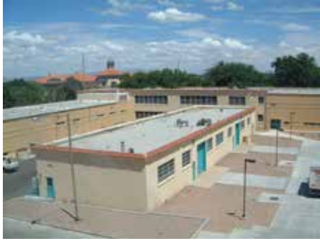
Photo taken in March of 2001 from the third floor of Engineering Complex 3.
