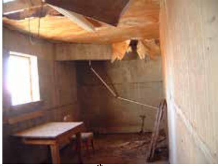
Room on the 5 th floor of the tower.
