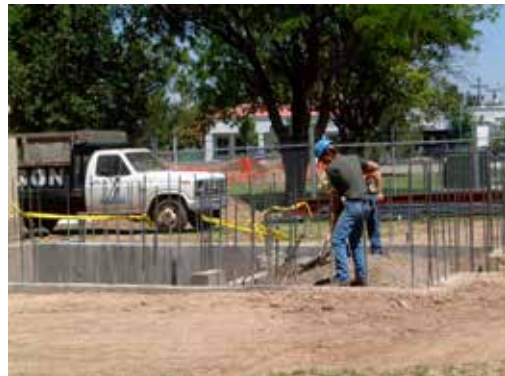
Digging the footing for the new elevator shaft.
