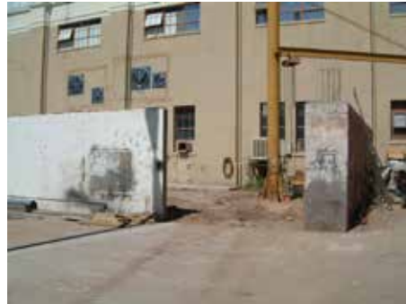
West side of the building.
