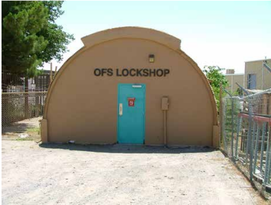
West side and main entrance to the Lock Shop. Photo taken June 11, 2004.
