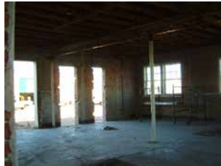
Looking northeast in the kitchen area.
