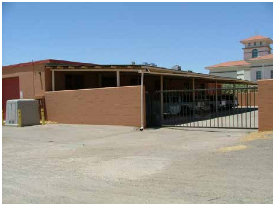
Photo of the southeast side of the building taken June 11, 2004.
