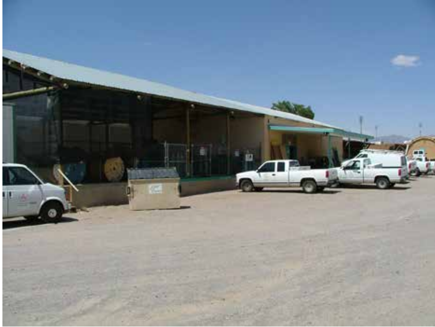
South side of the building. Photo taken June 11, 2004.
