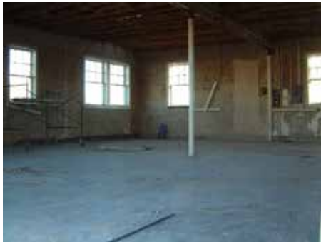
Looking southeast in the kitchen area.
