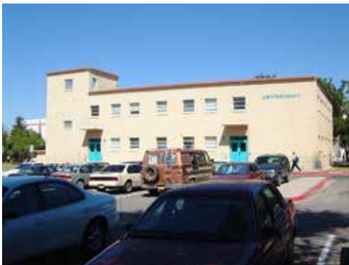
South side of the building. Photo taken September of 2000.
