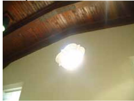
Inside the main lobby: window above the main entrance.
