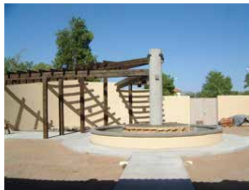
New enclosed patio area on the north east side of the building.
