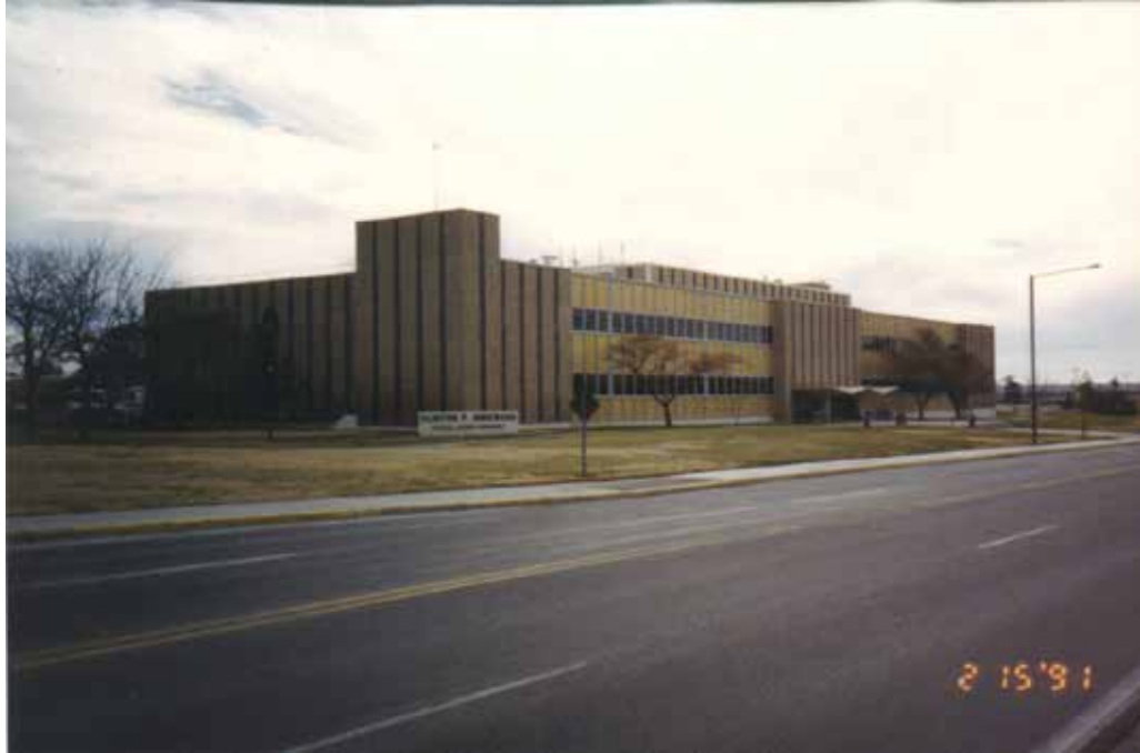
Photo of the north side of PSL before its renovation. Photo taken February 15, 1991.
