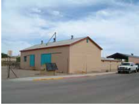
Photo of the northwest side of the building taken April 27, 2004.
