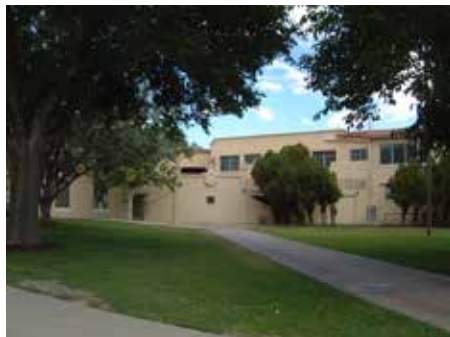
West side of Milton Hall. Photo taken May 25, 2001.
