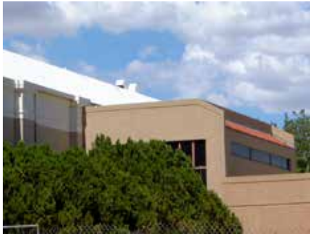
West side of annex connection to the main building.
