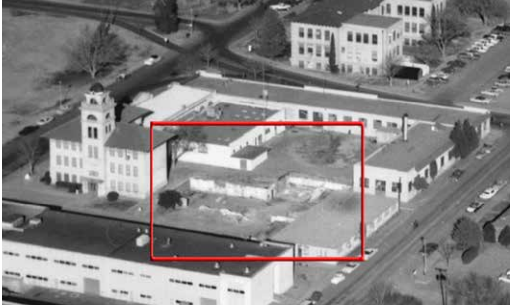
Photo showing the remains of the old steam plant after demolition in 1968. Photo courtesy of University Archives.
