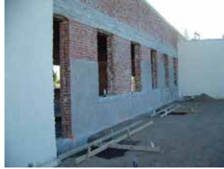
Northern exterior wall of the dining area.
