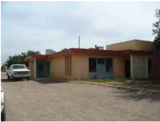
Front of the Livestock Office. Photo taken April 27, 2004.
