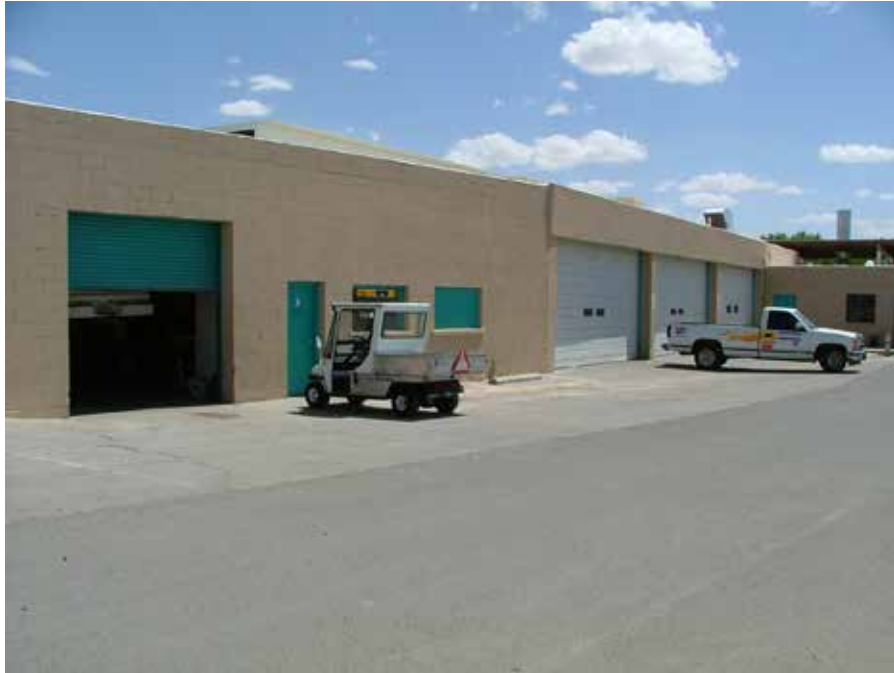
South wing of the shops building is home to the mechanic's shop. Photo taken June 11, 2004.
