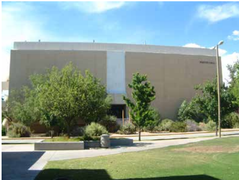
South side of Foster Hall. Photo taken July 14, 2004.
