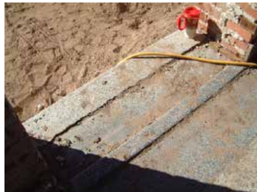
South entrance threshold.
