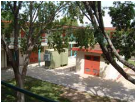
East courtyard and pump house.
