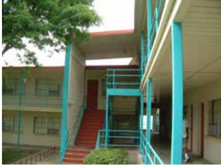
Stairs on the northwest side of the southeast wing.
