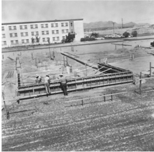
Construction photo from 1962. Photo courtesy of University Archives.
