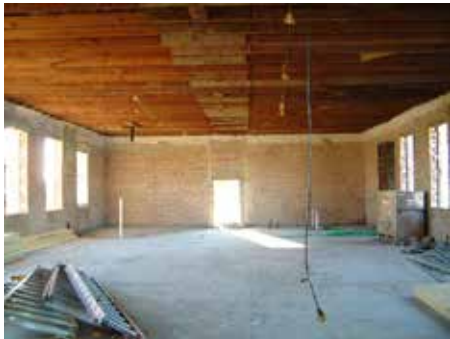
Looking west in the dining area.
