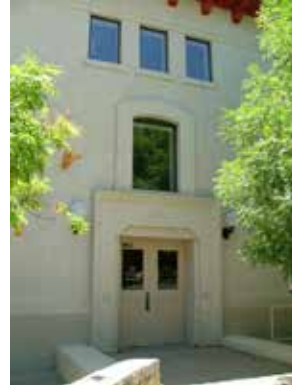
East entrance to the building. Photo taken June 11, 2004.
