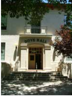
Front of Dove Hall. Photo taken June 11, 2004.
