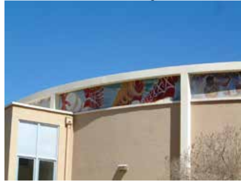
This musical mural is a tell tale sign of the buildings original use.
