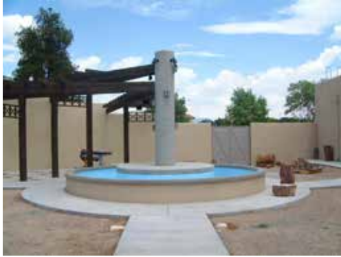
The fountain still under construction.
