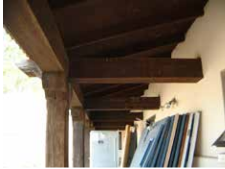
Rafters for the back porch.
