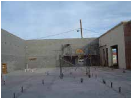
The new addition with concrete slab laid.
