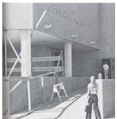
Photo from the 1977 yearbook. Photo shows the re-enforcing supports on the building while efforts were made to prevent the building from "sinking".
