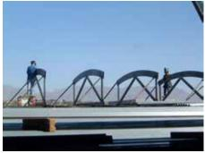
Working on the very top of the building, workers are welding on these steel trusses.
