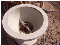
The Urns that are found on the corners of the tower. Appears to have once held electrical outlets for lighting, etc. The urns measure 3' in diameter and 2.5' in height.
